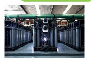
UF membrane racks in Qindao desalination plant
